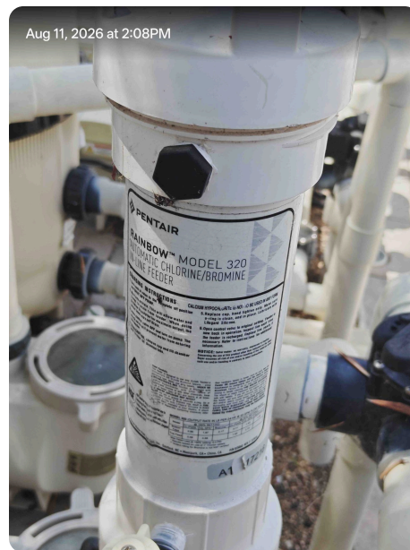
Sanitizer S-2: second Pentair Rainbow Model 320 in-line chlorinator.
