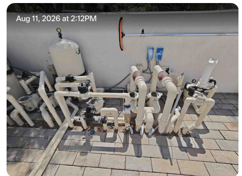
Supporting site photograph 32.
