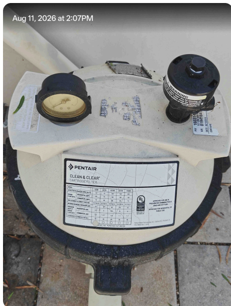
Filter F-2: Pentair Clean & Clear CC50, manufactured June 2019.
