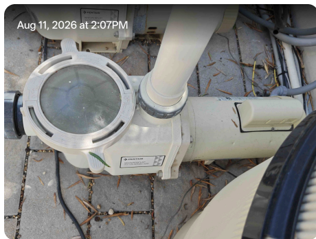
Pump P-4: Pentair WhisperFlo High Performance pump.
