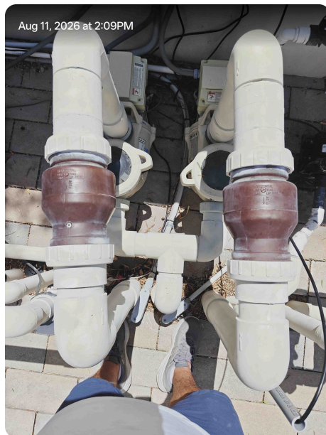
Supporting site photograph 18.
