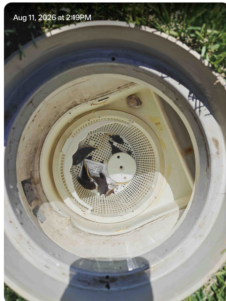
Supporting site photograph 39.
