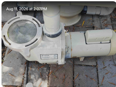
Pump P-5: Pentair WhisperFlo High Performance pump.
