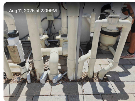
Supporting site photograph 21.
