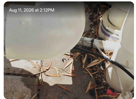
Supporting site photograph 30.
