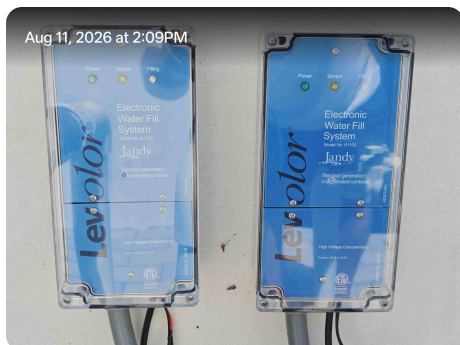
Two Jandy Levolor K-1100 electronic water-level controllers.
