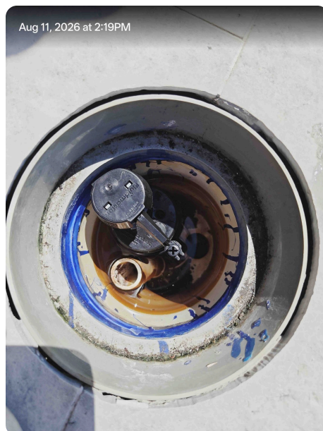
Supporting site photograph 40.
