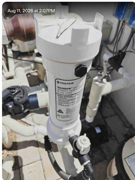
Sanitizer S-1: Pentair Rainbow Model 320 in-line chlorinator.
