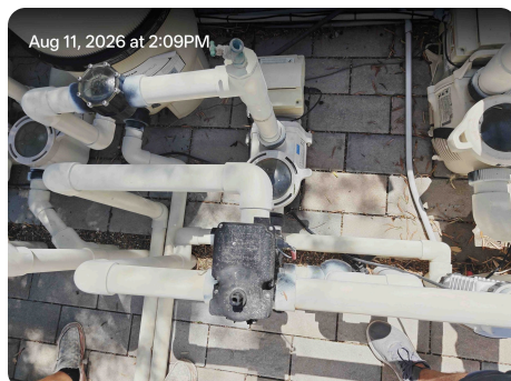
Supporting site photograph 19.
