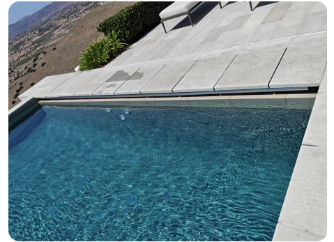
Pool overview showing the existing calcium line at the waterline.
