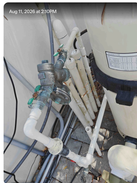
Supporting site photograph 23.
